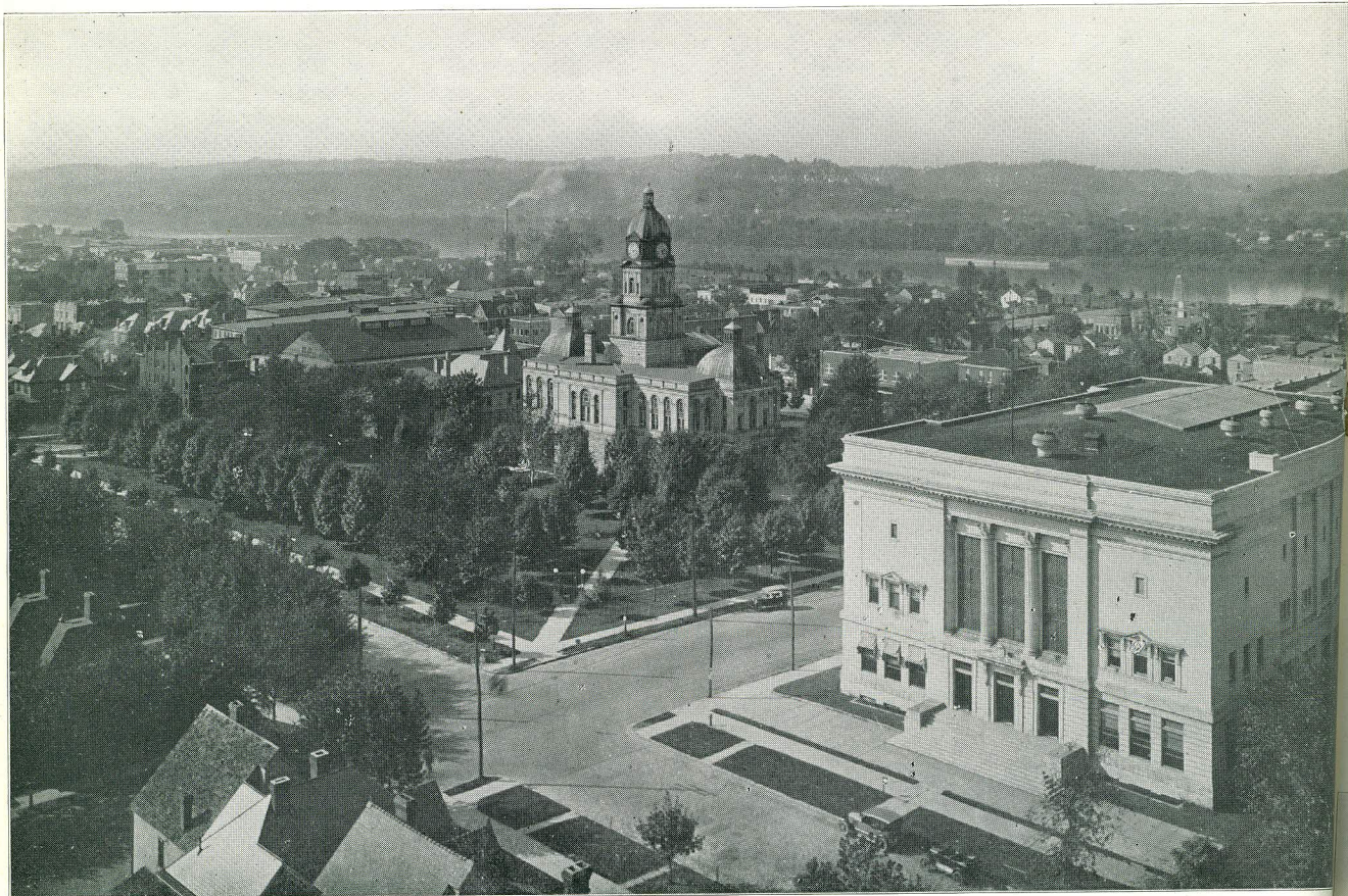
FROM ROBSON-PRICHARD BUILDING, SHOWING CITY BUILDING IN RIGHT FOREGROUND
