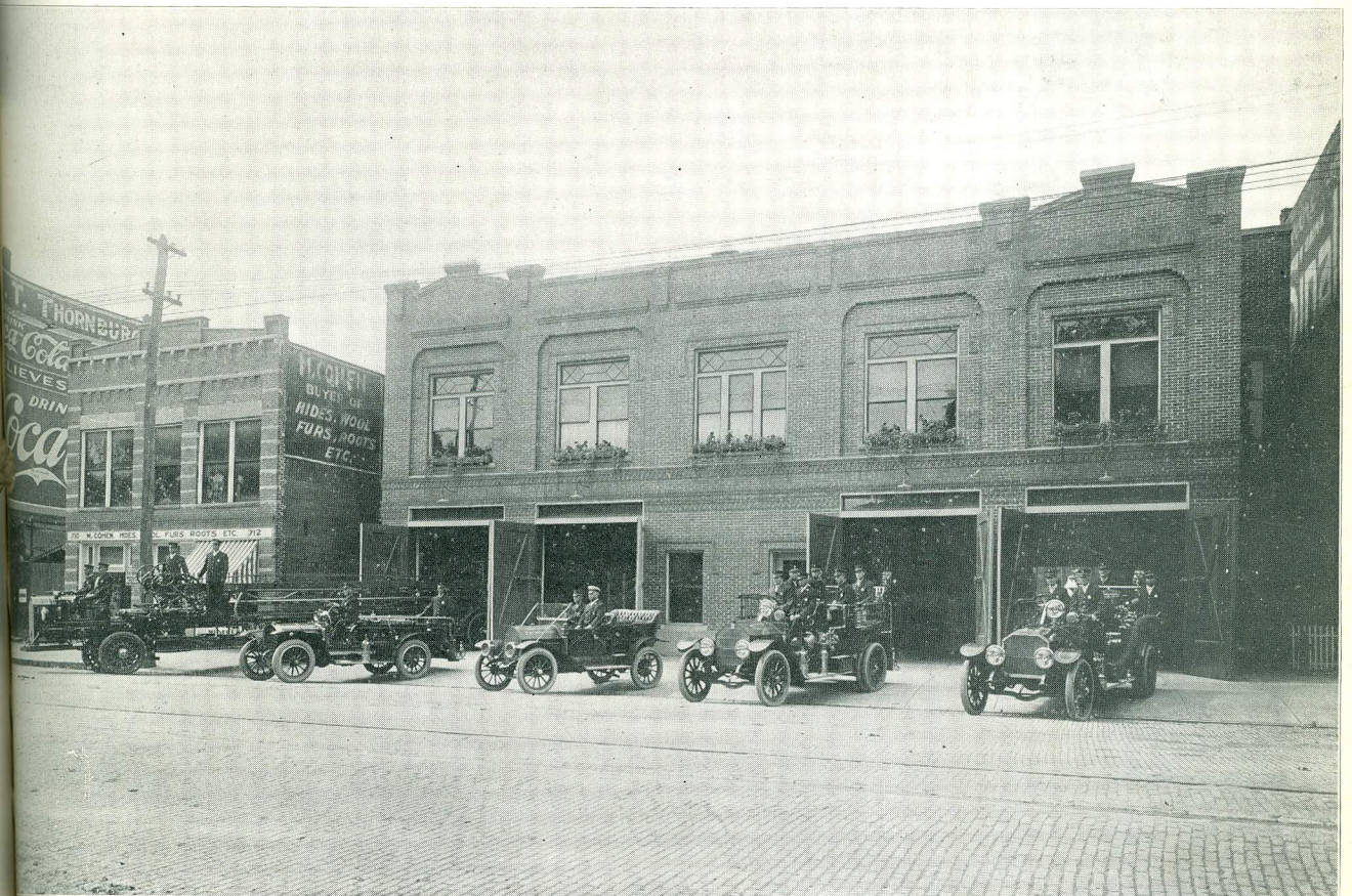
CENTRAL FIRE STATION
