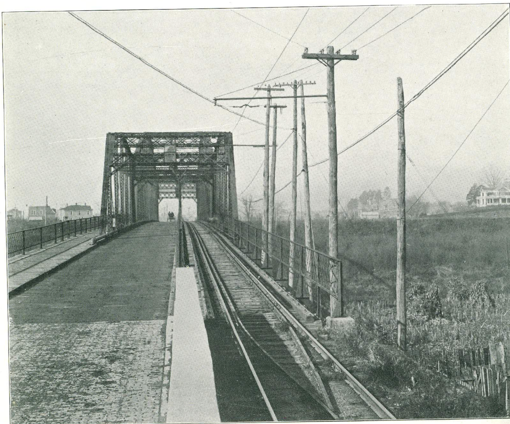
THE NEW GUYAN BRIDGE
