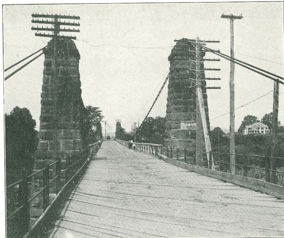
OLD BRIDGE ACROSS GUYAN RIVER
